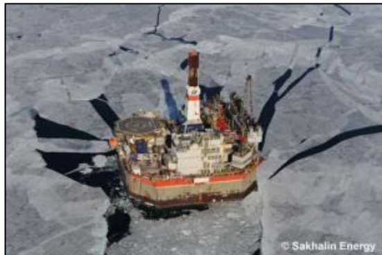
The Molikpaq platform, February 2009, Sakhalin-2 project, courtesy Sakhalin Energy
