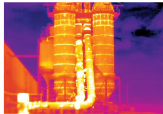
Infrared Inspection of Petrochemical Plant
