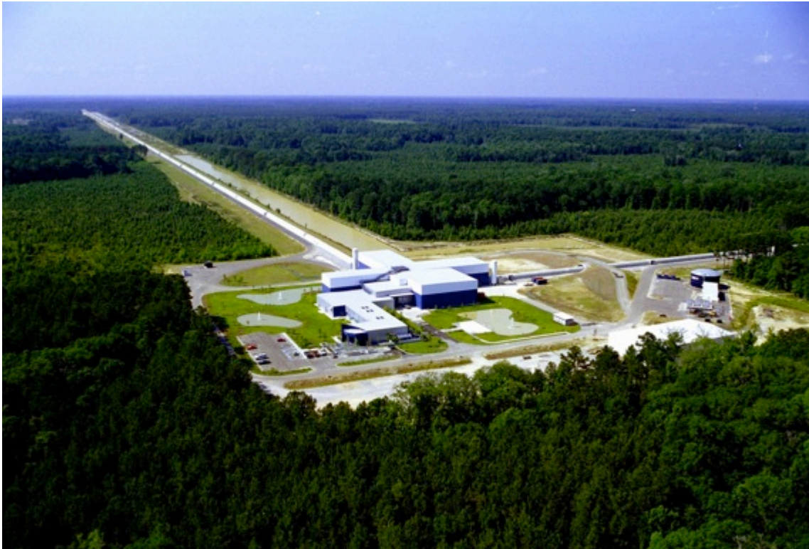
The 4 km arm length LIGO gravitational wave observatory in Louisiana, part of the world-wide effort to detect gravitational waves
